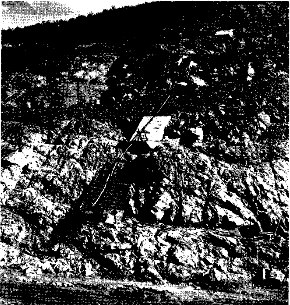
Figure 11.1. Abutment of Dartmouth Dam showing cleanup in cutoff foundation, and construction of the grout cap (courtesy of Rural Water Commission of Victoria).
