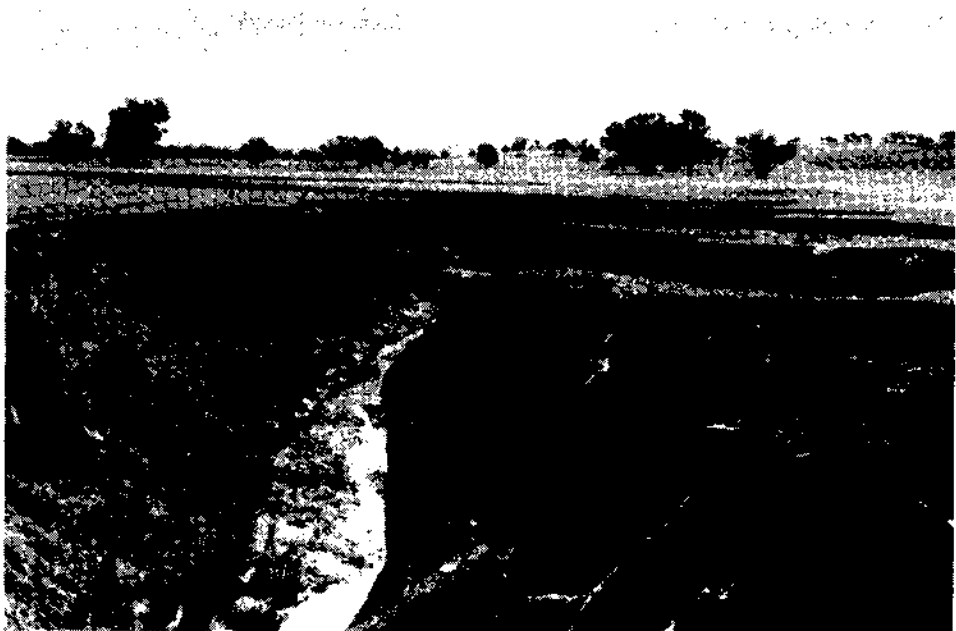
Figure 8.24. Deep erosion gulying in dispersive soils (Soil Conservation Service of NSW).
